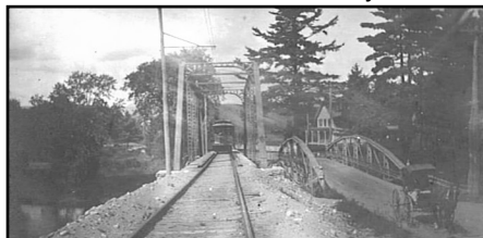
Plank Road Bridge.
