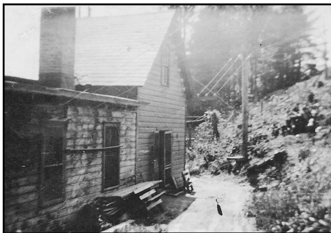
Smith Electrical Building See also two photos on page 5
